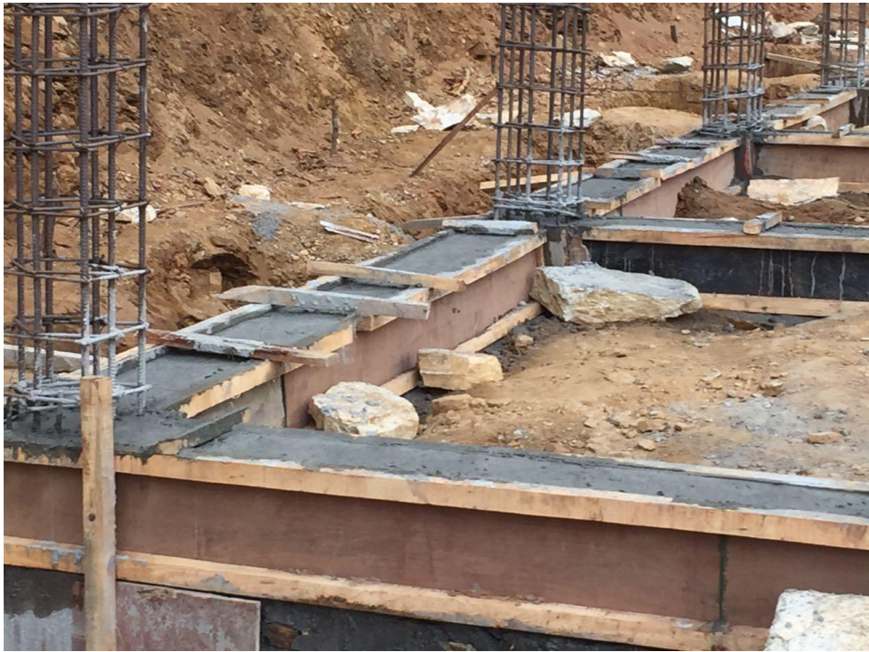
CONCRETING OF PLINTH TIE BEAM
