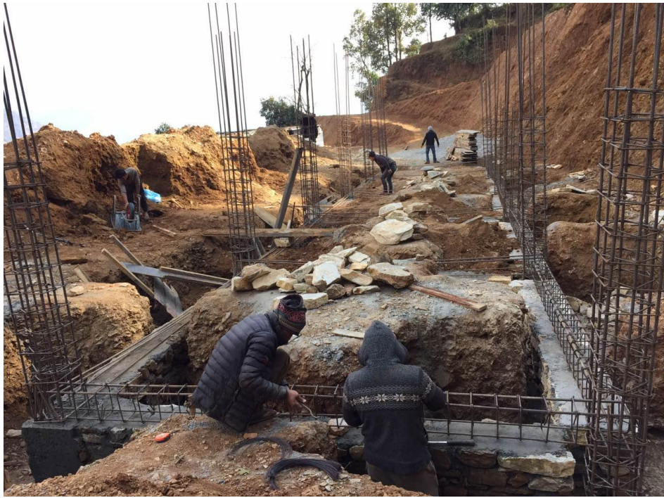
FOUNDATION FILLER WALL AND PREPARATION OF PLINTH BEAM
