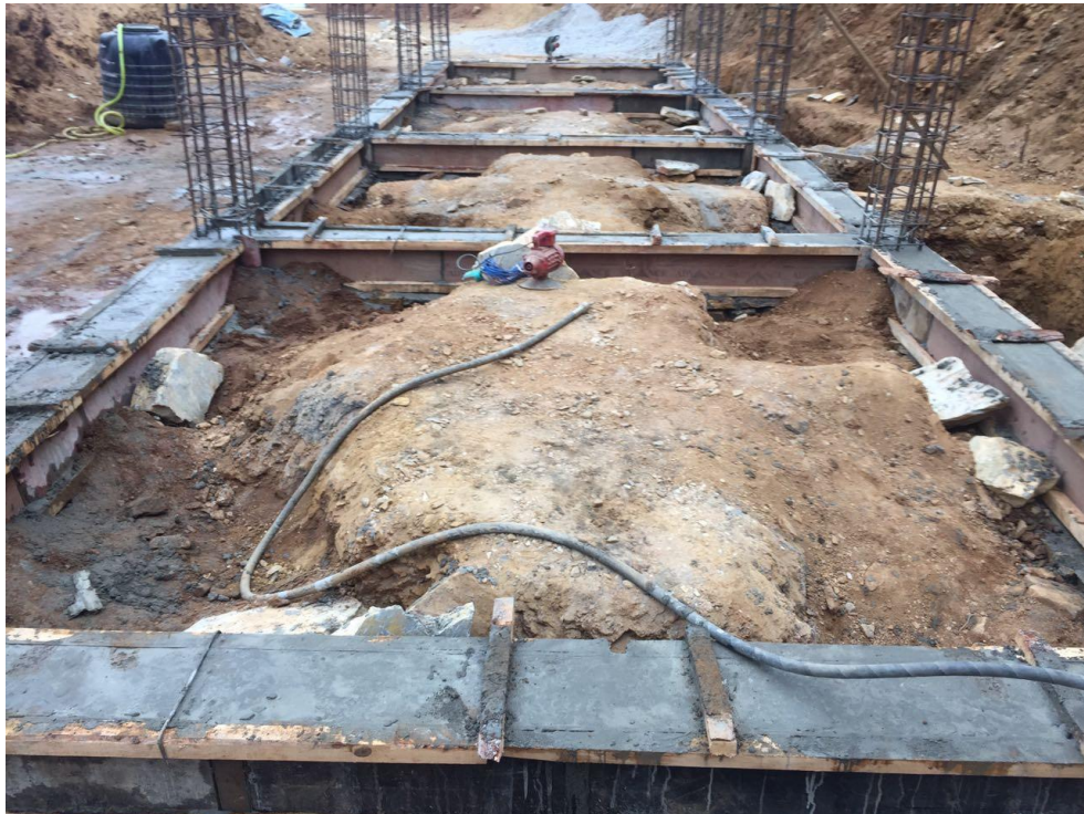
COMPLETION OF PLINTH STAGE OF BUILDING
